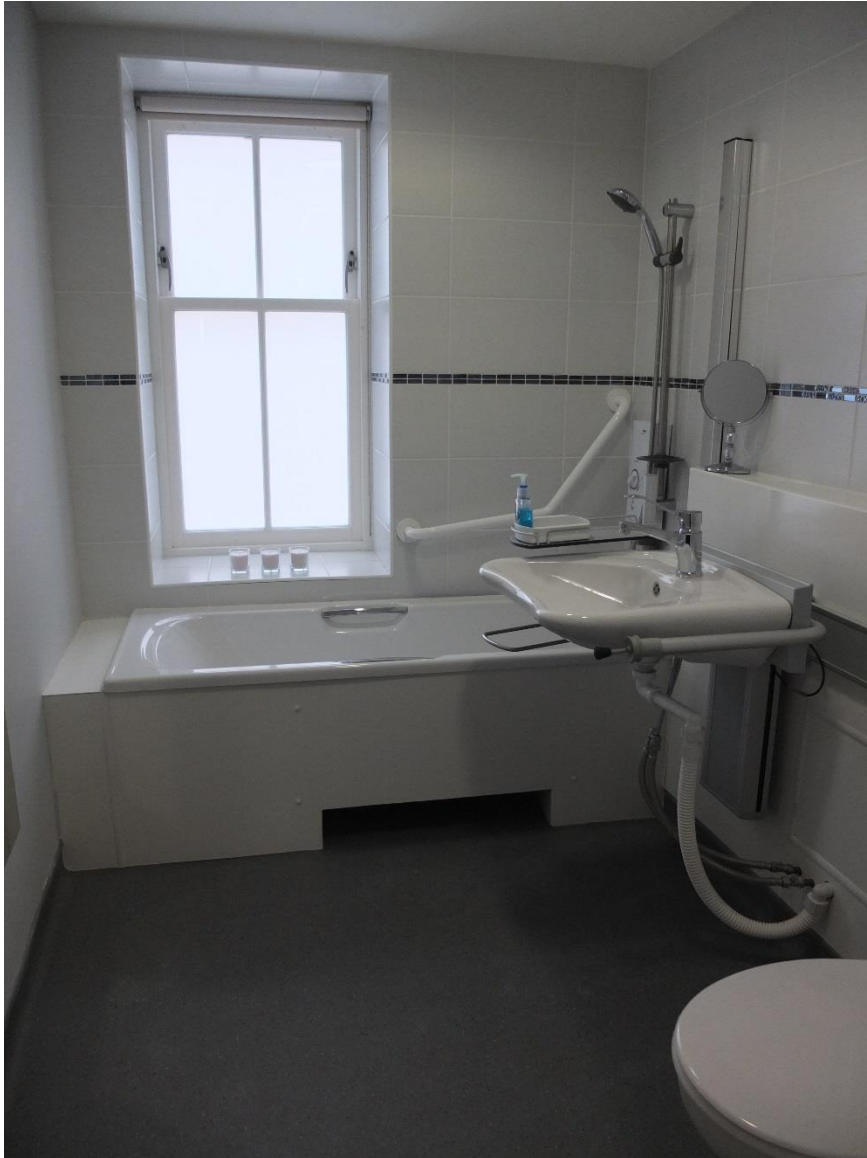
Image: Bath with adjustable sink and toilet.
