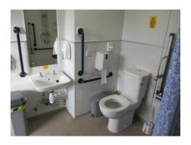
Within Toilet Blocks 1 and 2 **male and female toilet** doors achieve an 800mm clear opening width over a level threshold. Ambulant disabled WC and shower cubicles are provided with contrasting grab rails. Showers are level access with a recessed drainage gulley. WC's, basins and showers have ergonomic lever style controls.
